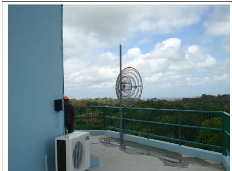
Bottom row: Left: Microwave transmission of data to Meteorological office
